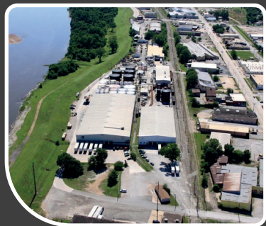
Grease Lubricant Plant Tulsa, Oklahoma
